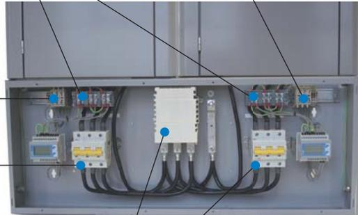
250A rated main supply      Independent 125A protection device for each board supply
