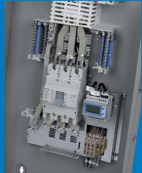
Eaton's unique solution uses smart meter technology to monitor embedded transducers in a high integrity shrouded 200A busbar assembly. This solution provides independent readings of each section of the board as net values, as well as providing information of the total demand on the board – all from a single smart meter.
