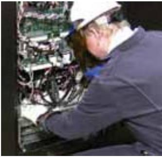
The 9395s modular design lets service technicians disconnect one UPM while the remaining UPMs support the load.
