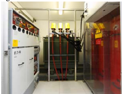
Figure 1 Medium-Voltage cubicle
