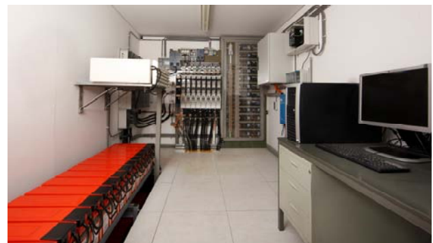
Figure 2 Low-Voltage cubicle
