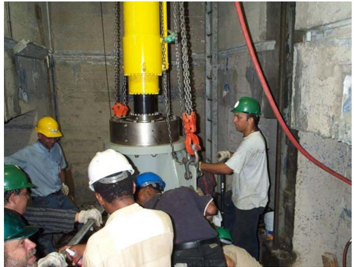
the canal's rising stem valves, which control water flow through the culverts. Each unit has a redundant-style, dual 30-horsepower electric motor pump grouped with Eaton's new Series PVM050 load-sensing, pressure-compensated 50cc variable displacement piston pumps.
