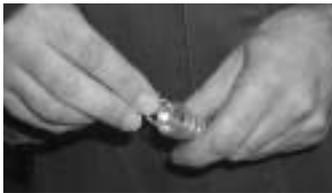
**Figure 5 - Braze ring installation**
