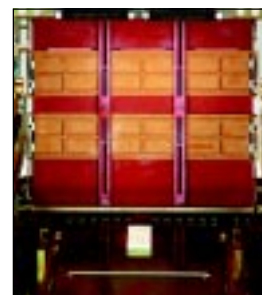
The independently operated and lockable shutter design provides a safe environment when the breaker is removed from the cassette.
