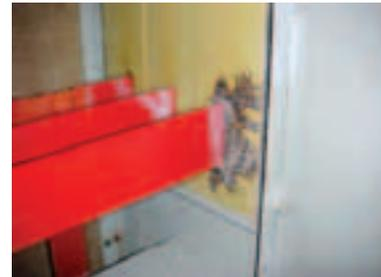
*PD Between Bus and Cubicle Wall*
