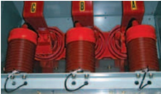
*An Example of Installation of a Set of Coupling Capacitors*
