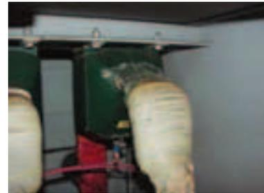
*PD Damaged Insulation on Current Transformer*
