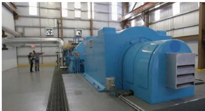
New turbine room with 19.8 MW steam turbine-generator. (Photo courtesy of *The Register-Guard*)
