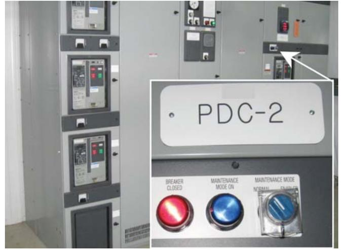
The new front-accessible low voltage switchgear assembly for PDC-2 is shown above. The main circuit breaker includes a lockable Maintenance Mode Switch and a blue indicating light. The switch can be locked in the NORMAL or the ENABLED mode. In the ENABLED mode, the blue light is illuminated and the breaker responds to the instantaneous maintenance setting.
