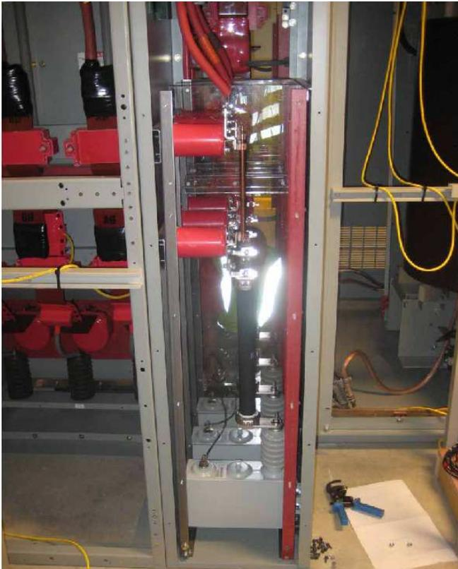
Figure 15. RC Snubber (Typical Installation for this Facility)
