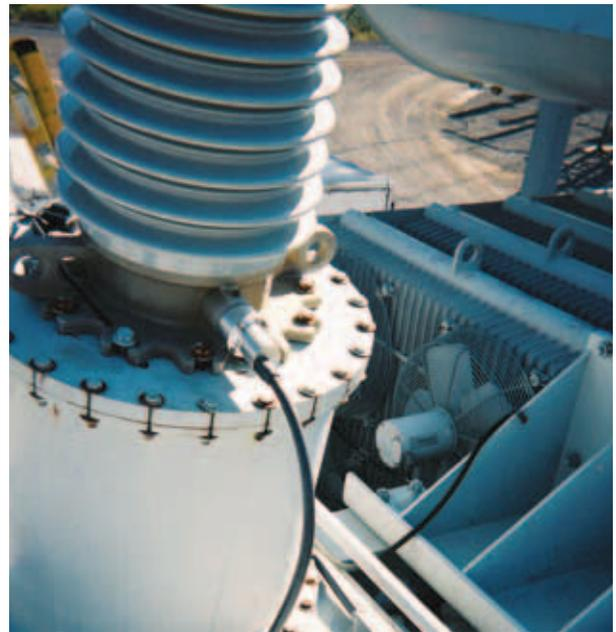
*Sensor installed in capacitor tap on bushing*
