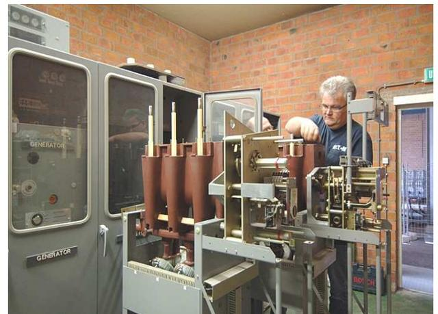
Fig.1 Maintenance of 30 years old minimum-oil breaker.
