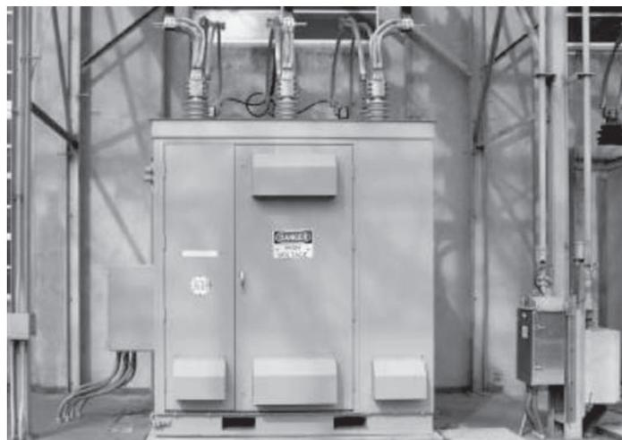
**Figure 10. Installed Vacuum Circuit Breaker (Photo Courtesy of Southern Company)**
