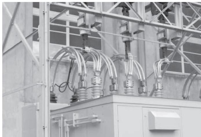
**Figure 9. Circuit Breaker Bus Connections (Photo Courtesy of Southern Company)**
