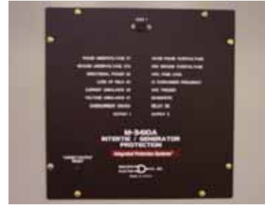
Figure 7. Protective Relay
