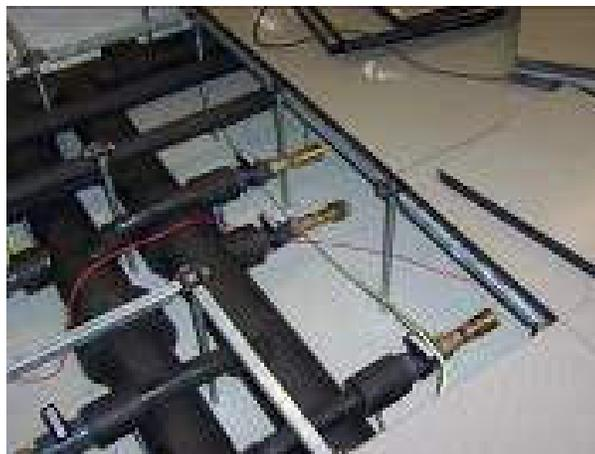
*Figure 3: Under floor or overhead piping with quick connects can be added during initial construction, though they can increase construction costs.*
