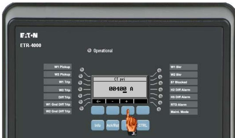
Enter the desired CT setting using the soft keys. When the appropriate setting is displayed, follow the same procedure to change the setting:
