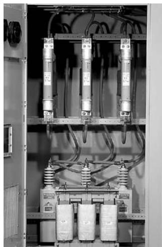
Harmonic filter capacitor stage enclosure
