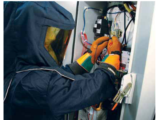
Worker wearing PPE
