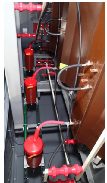
38 kV coupling capacitors installed at a dry-type transformer terminals
