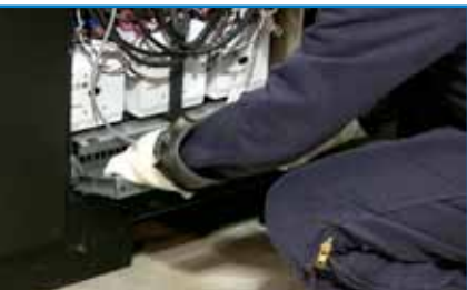
The 9395s modular design lets service technicians disconnect one UPM while the remaining UPMs support the load.
