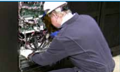
The 9395s modular design lets service technicians disconnect one UPM while the remaining UPMs support the load.
