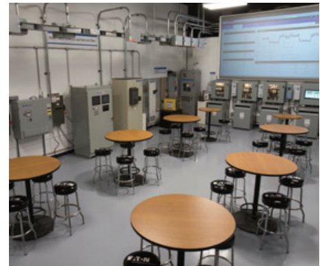
Power quality lab
