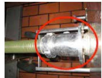
**Fig. 8:** Incorrect, unsuitable extension piece
