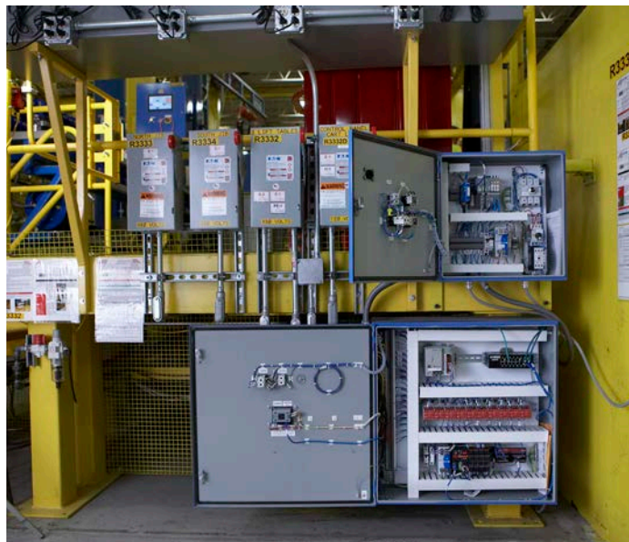
Figure 7.6.5.a Existing installation labeling per 240.86(A) and 110.22(B).
