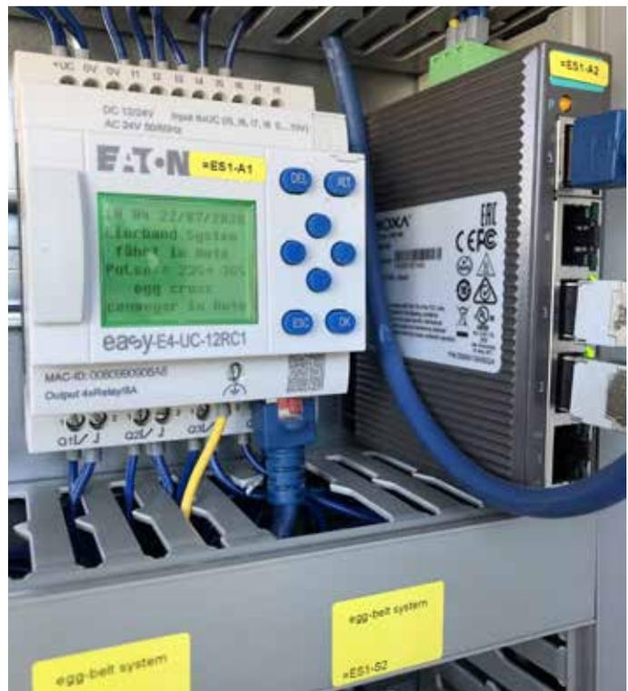
switch on the master control cabinet is used to select the hen house in which the conveyor should operate. An M22 signal lamp, also from Eaton, which is located above the conveyor indicates whether the eggs from a hen house have already been collected, are currently being collected or if a fault has occurred.
