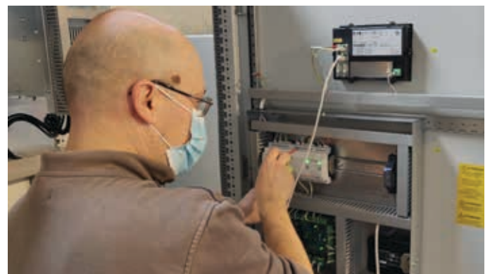
The easyE4 enables equipment to provide accurate information about the entire system. The data collected is transferred to the cloud in order to monitor the condition of the machine or for preventive maintenance.
