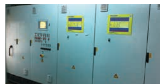
The operation of the system may be either fully automated using Eaton's control system, or it may be operated manually using a Neuero switchboard
