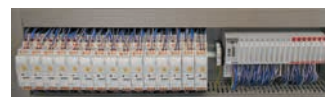
At Neuero, the EMS is primarily used as a reversing load relay with integrated motor protection
