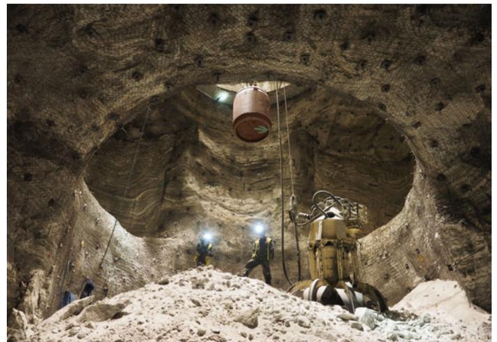
Deilmann Haniel plans to complete the construction of shafts in 2017 and produce its first ore in 2020. The new mine will have two shafts: a 465-meter deep shaft with skip winding (for hoisting the ore) and a shaft with cage winding (for hoisting and descending workers and loads). The mined ore will be processed at the Berezniki-3 plant, where a 6.3 km cable-belt conveyer will transport it.
