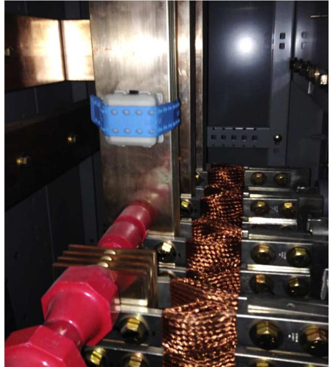
Fig. 9: Acoustic sensor attached to energized bus bar in low-voltage metal-enclosed switchgear.
