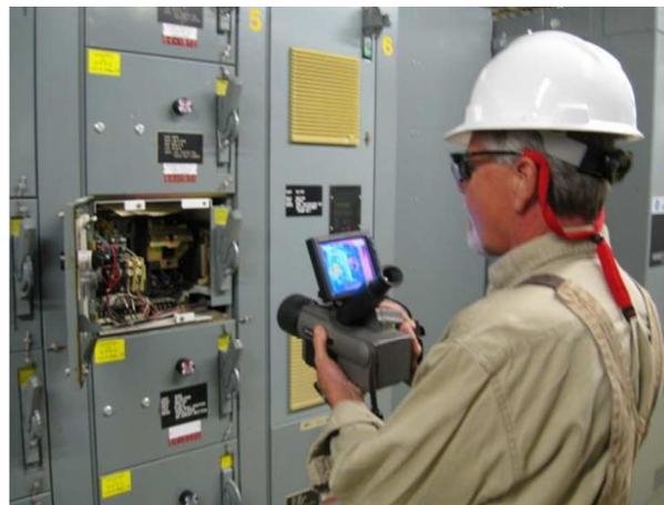
Fig. 2: Thermographer conducting an IR scan of a low-voltage motor control center unit with the unit door open.
