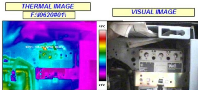
Fig. 1: The thermal image at left shows an elevated temperature and possible loose connection at the Phase A line terminal of the circuit breaker
