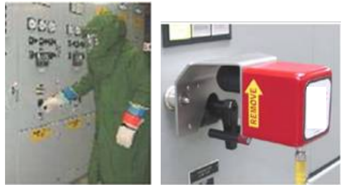
Figure 12. Local switching (Left) vs. Remote switching (Right)
