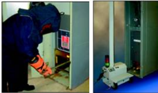
Figure 10. Conventional Racking (left) compared to Robot (right)
