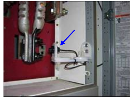
Figure 20. Remote Temperature Sensing
