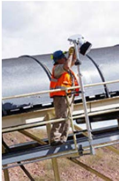
Fig. 4: Telescoping light poles being installed in mine site conveyor system
