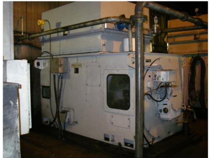
Fig. 7: 6,000Hp Dryer Exhaust Fan Wound-Rotor Motor
