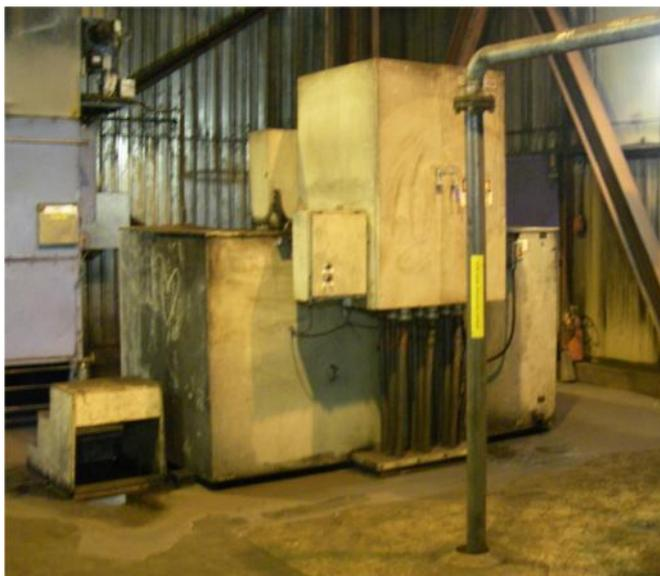
Fig. 8: Existing liquid rheostat for 6,000Hp motor which was decommissioned as a part of the VFD upgrade
