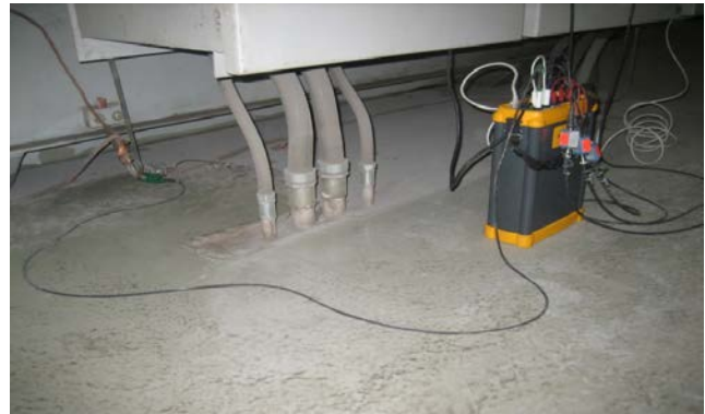
Figure 3. (a) The voltage dividers installed at LMF1 primary, (b) The transient recorder and grounding for LMF1
