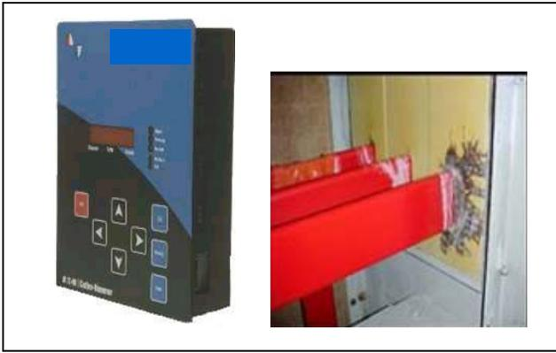
Figure 18. Partial Discharge Relay and Switchgear with Pending Failure
