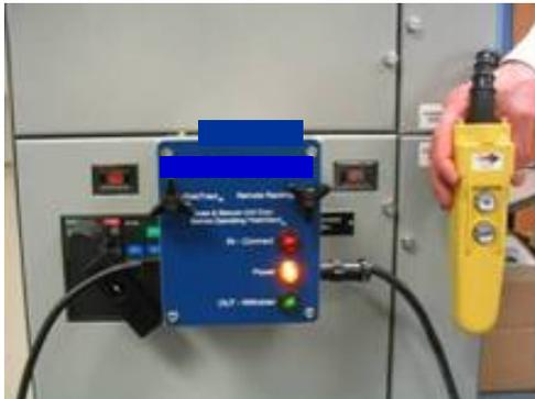
Figure 11. New LV Motor Control Center with Remote Racking Device
