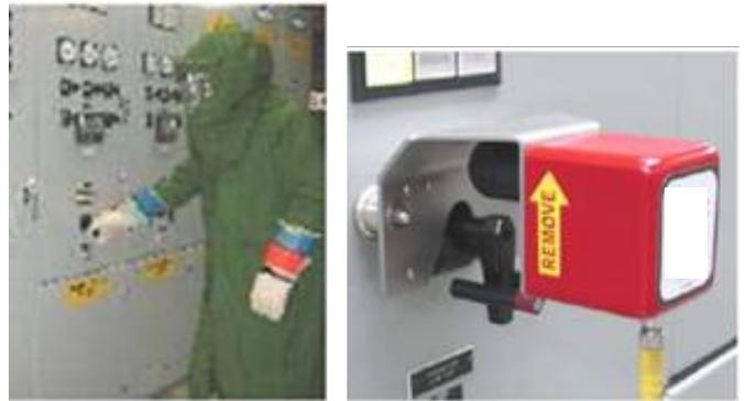
Figure 12. Local switching (Left) vs. Remote switching (Right)
