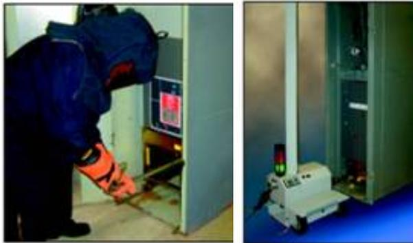
Figure 10. Conventional Racking (left) compared to Robot (right)
