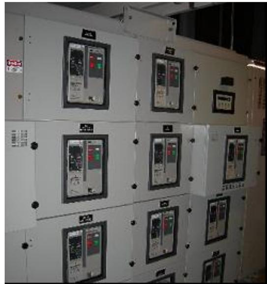
Figure 5. Retrofilled Fuses with Breakers Example
