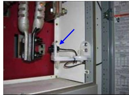
Figure 20. Remote Temperature Sensing
