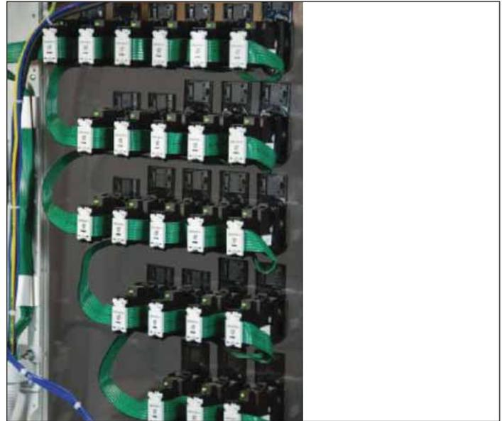
**Figure 6. Device-level wiring systems use flat multiconductor cables to connect components, replacing bulky wiring ducts found in conventionally wired control panels**
