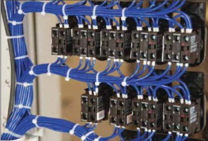
**Figure 2. Additional control panel construction time is required when wiring is bundled to door-mounted devices because wires must not restrict opening and closing the door**
