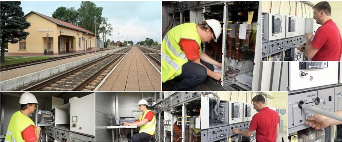
Eaton Xiria ring main units and SVS 08 series switchboards for the project. Another key factor was the very compact construction of these products, which not only made them easier to handle, but also meant that they could be accommodated in smaller buildings with lower construction costs.
