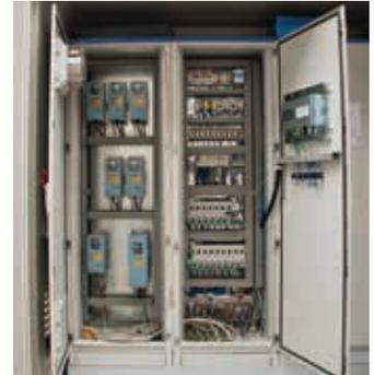
The Eaton SLX9000 inverters are communicating with the PLC via CANopen; motor starters are connected to the PLC via SmartWire-DT.
