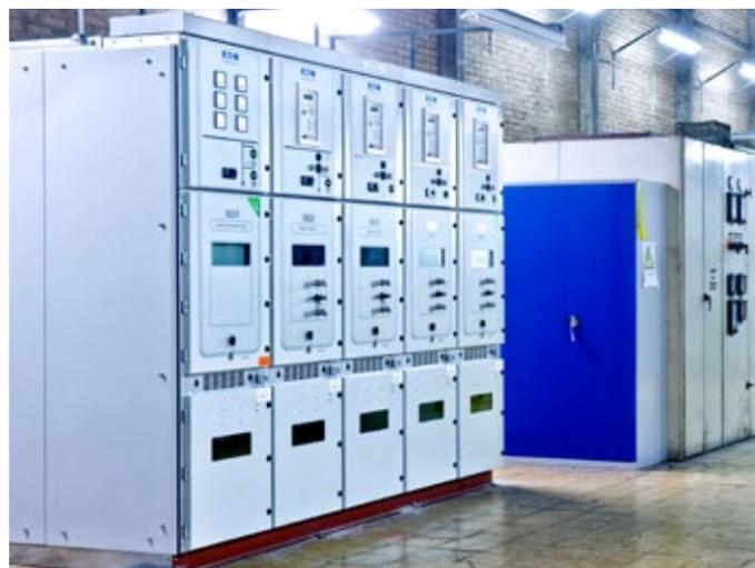
Power Xpert® UX, a safe and reliable medium voltage switchgear system used at Tata Steel.
