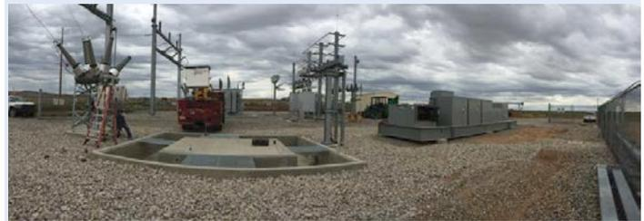
Jemez Mountains Electric Cooperative: installation of pad to house new transformer, new breaker installation, and MITS shown on right.
