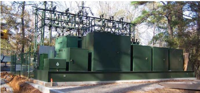
New Eaton modular integrated transportable substation (MITS) in front of open air substation to be retired shown behind.
