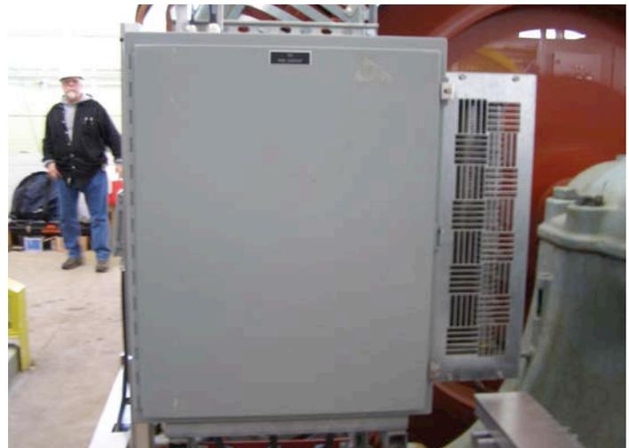
Small hydro high-resistance ground and generator neutral enclosure (hydroelectric facility in Maine)
