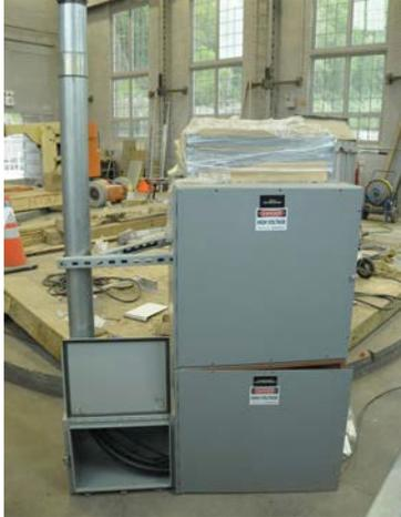
Combination generator termination cabinet (surge equipment) and high-resistance ground enclosure (hydroelectric facility in West Virginia)
