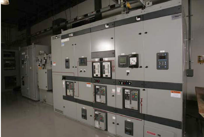
Low-voltage switchgear
