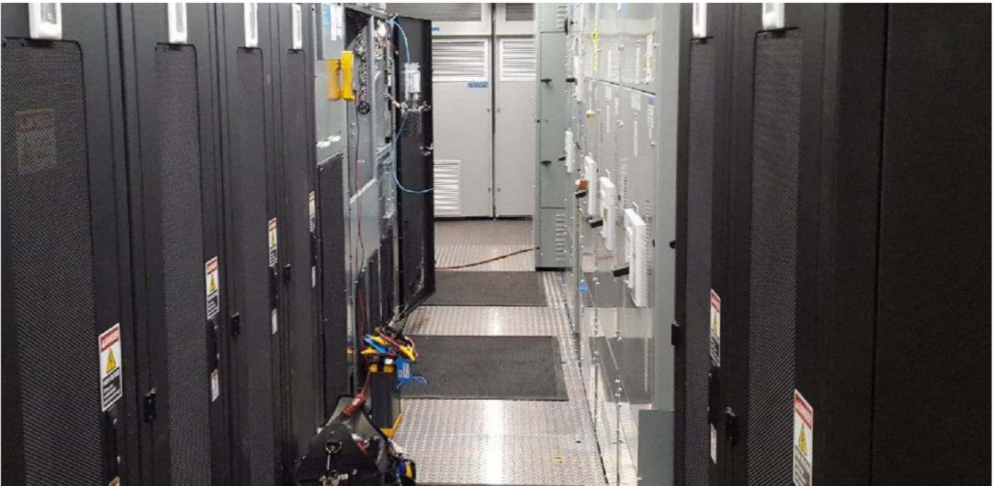
Power Xpert 9395 UPS with lithium-ion battery cabinets
