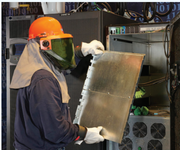
Proper preventive maintenance reduces the risk of UPS failure through thorough inspection, cleaning, testing and calibrating various electronic and mechanical components.
