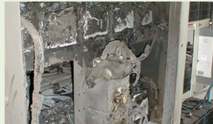
Thermal runaway effects on adjacent battery cabinet
