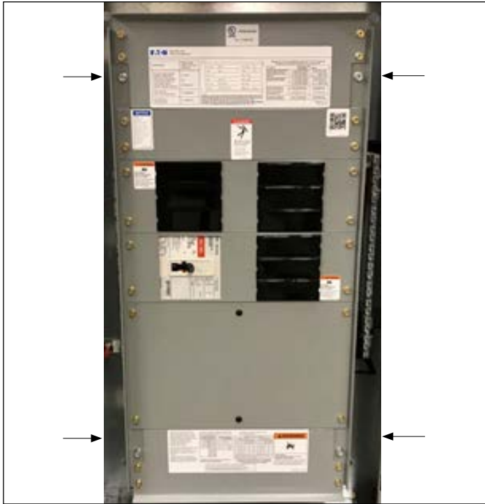
Figure 3. Remove panel and rails
