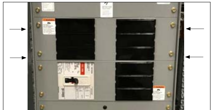
Figure 2. Remove panel
