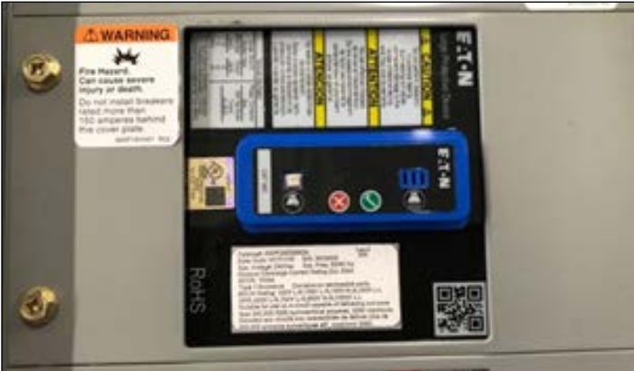
Figure 7. Apply label provided with SPD
