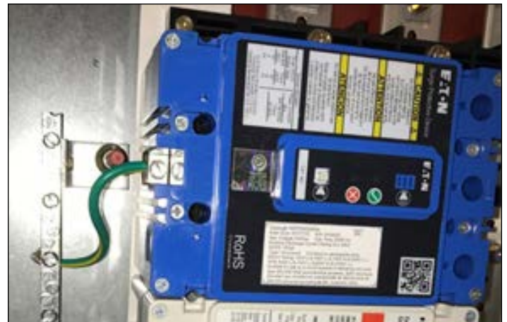
Figure 6. SPD installed—surge ground terminal
