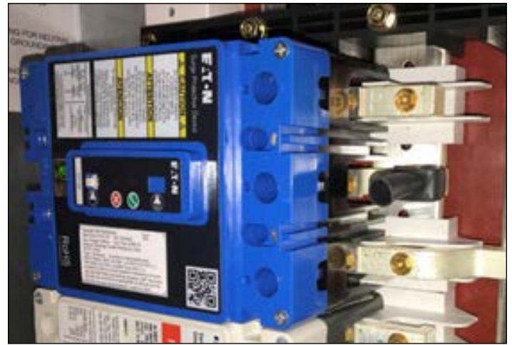
Figure 5. SPD installed—terminal side
