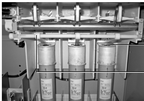
Blown Fuse Indicating Device
