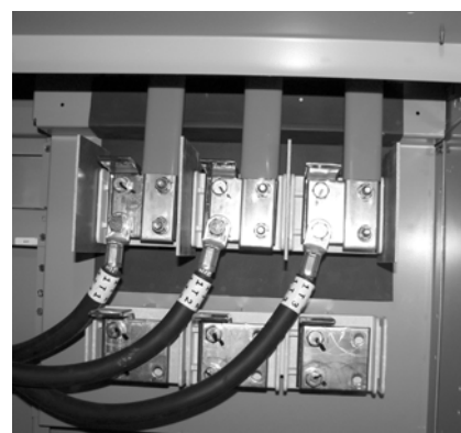
Load Cables—Moved for Full Voltage Start
