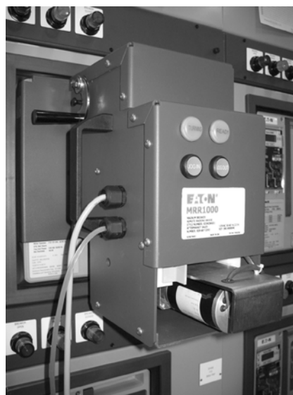
MRR1000 Connected to Magnum Breaker
