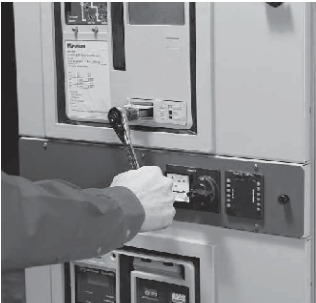
Figure 2-12 Levering position indication
