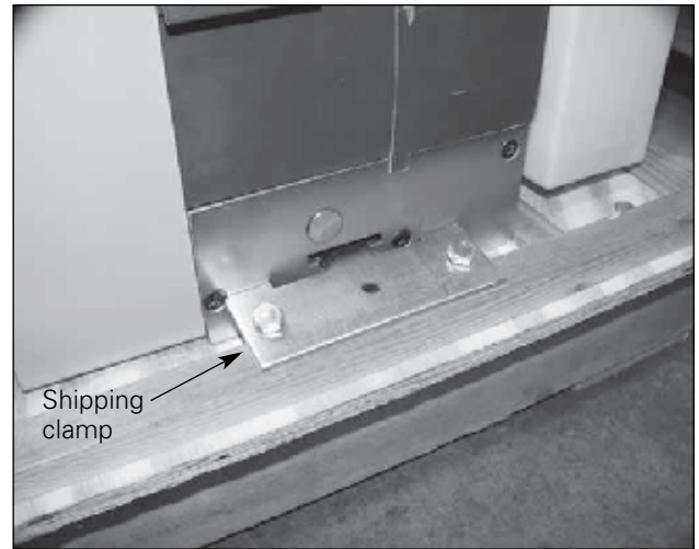
Figure 2-1 Shipping clamps for drawout circuit breaker
