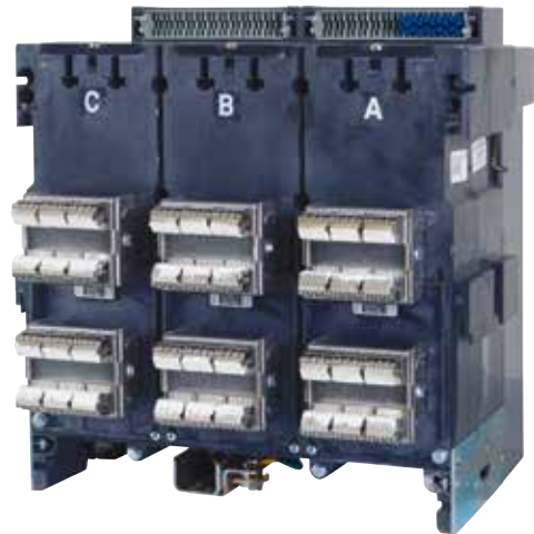
Figure 2-10 Drawout circuit breaker with automatic primary disconnects
