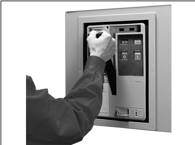
Figure 3-11: Circuit Breaker Closing Springs Being Manually Charged
