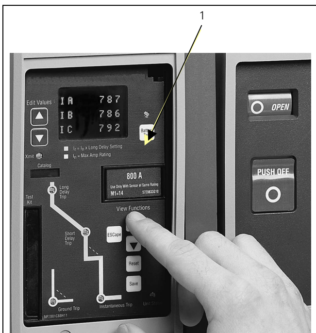
Figure 6-6: Trip Unit Rating Plug Location
