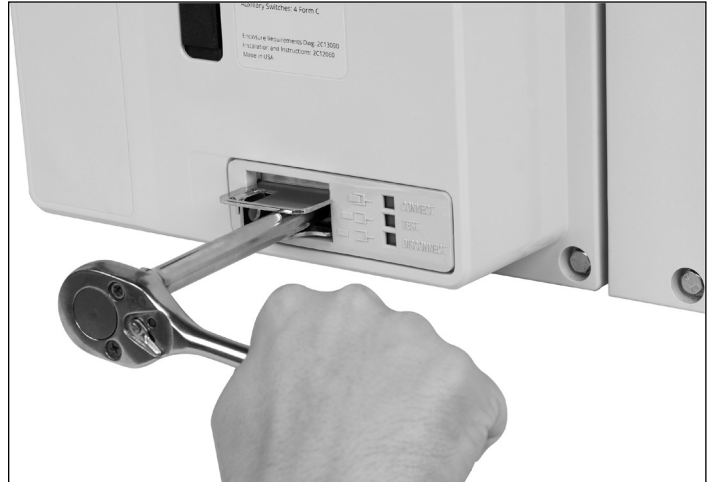
Figure 13. Levering position indication
