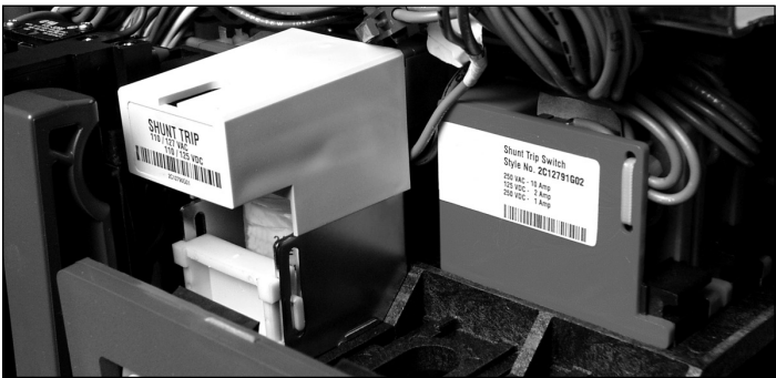
Figure 37. Shunt trip switch installed
