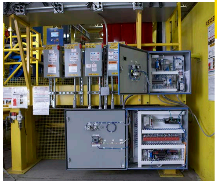
Figure 7.6.5.a Existing installation labeling per 240.86(A) and 110.22(B).
