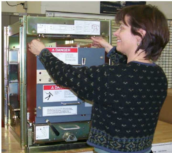
Figure 4: Put on or take off the dummy secondary cord bracket
